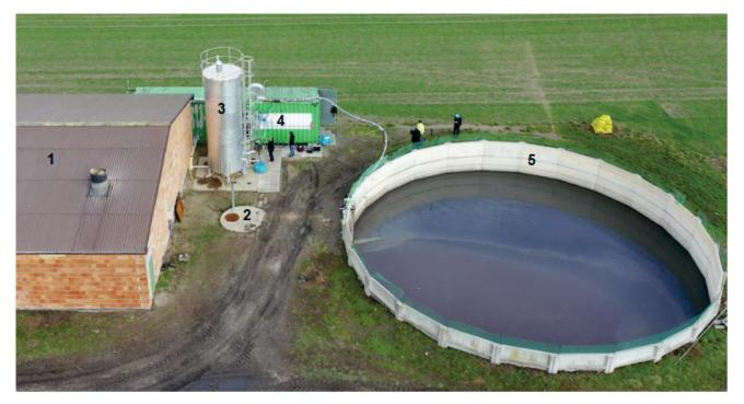
**Fig. 1.** Mobile pilot installation, example of the location of an agricultural biogas plant on a farm; I = livestock building, 2 = manhole to the well, the so-called "pre-tank for pig slurry", 3 = digester, 4 = container with the installation, 5 = digestate tank the so-called "lagoon"; souce: own elaboration
