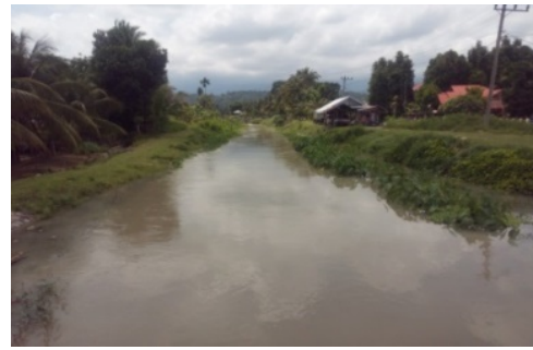
Photo 1. The condition of the structure, the primary channels of Baro Kanan (phot. A. Azmeri)
