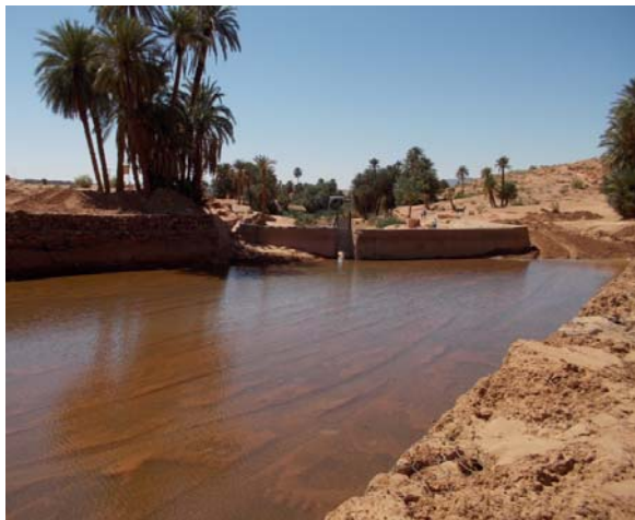
Photo 5. The ancestral Tiout dam is filled with water leaks (phot. B. Remini)
