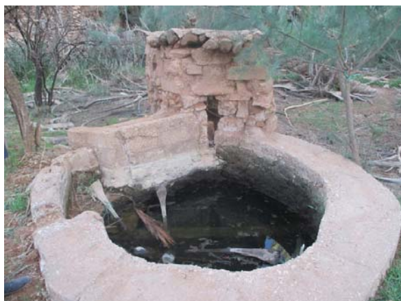
Photo 9. The water level is flush with the soil surface in a well of the oasis of Boussemgouhoun (phot. B. Remini)
