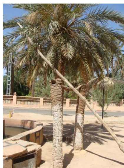
Photo 8. A pendulum well model at the entrance from the oasis of Moghrar Tahtani (phot. B. Remini)
