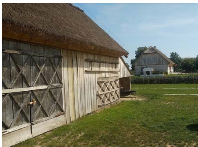
Photo 1. Traditional 'Olender' home with a lower level utility room that is periodically flooded and a boat used for travel and evacuation purposes; Antique building museum in Wiączemin Polski (Pol. Skansen Osadnictwa Nadwiślańskiego) (photo R. Mazur)
