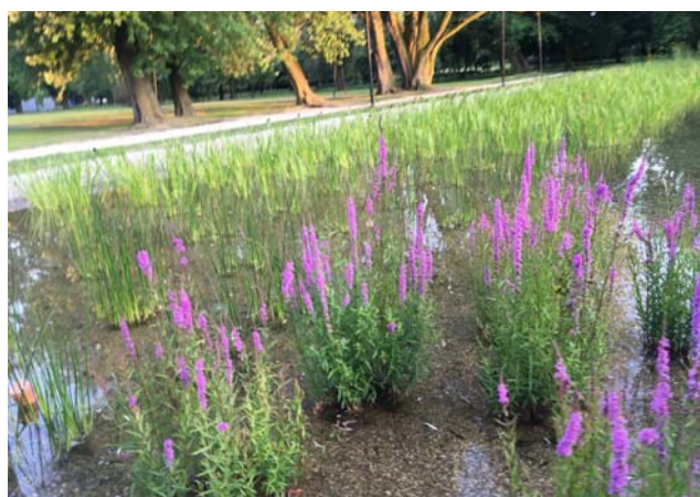
Photo 3. Mineral-plant filter with visible plantings of purple loosestrife, bulrush and calamus (photo: W. Walczak)
