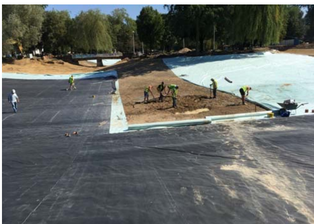
Photo 1. Profiling and sealing the bottom of the recreational reservoir (photo W. Walczak )
